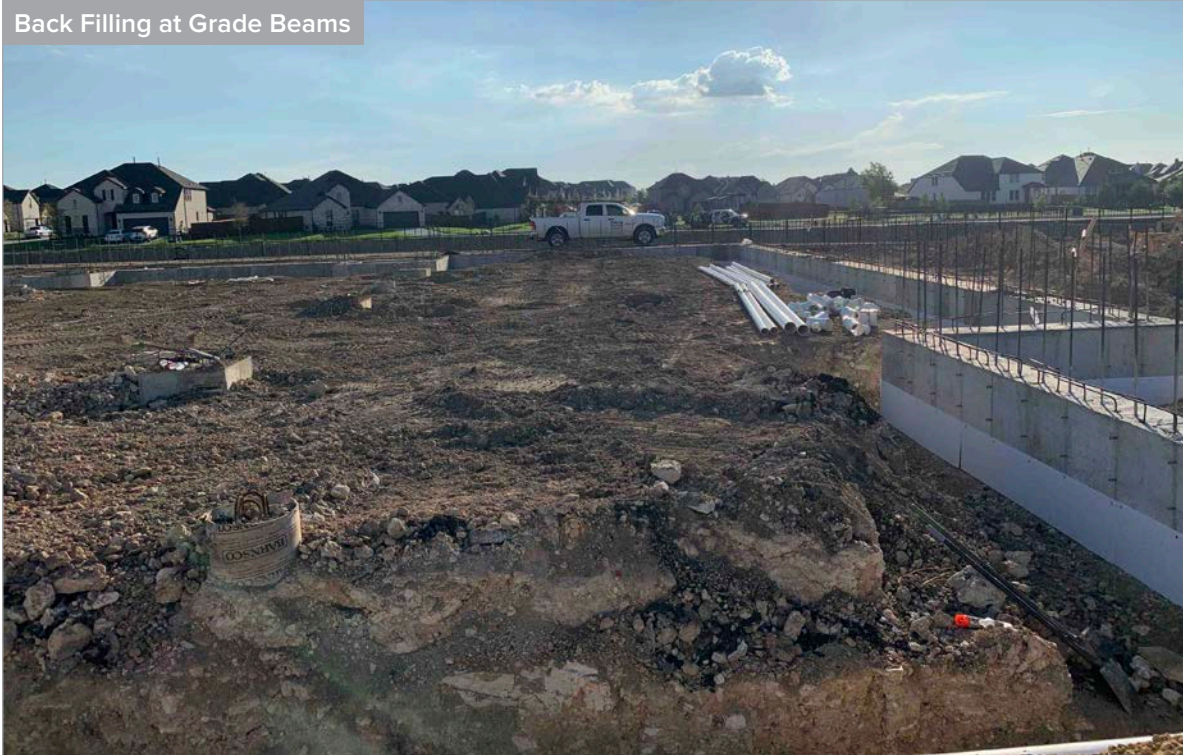
Preparing for Carton Form Placement
