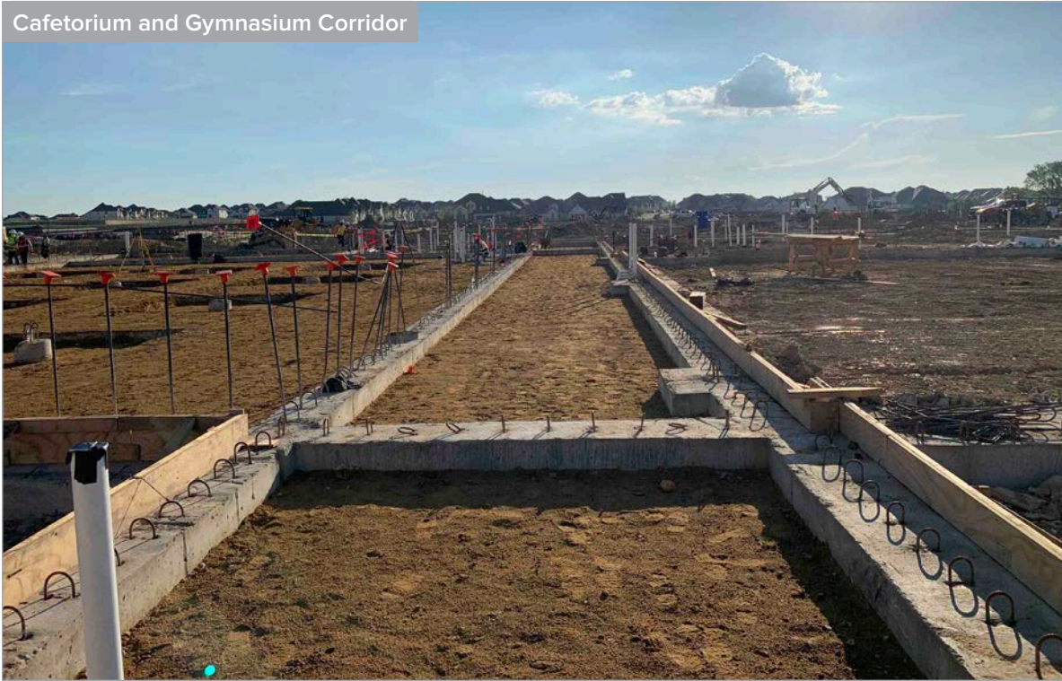
Underslab Plumbing at Kitchen Area
