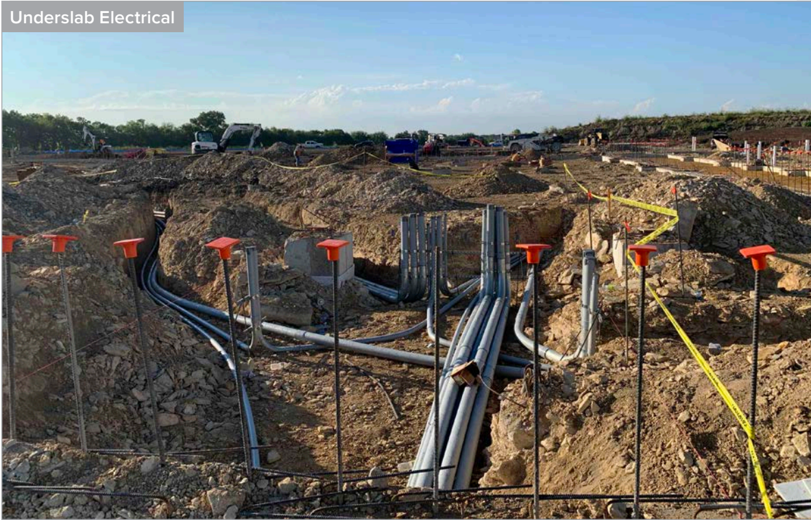
Underslab Electrical at Main Electrical Room
