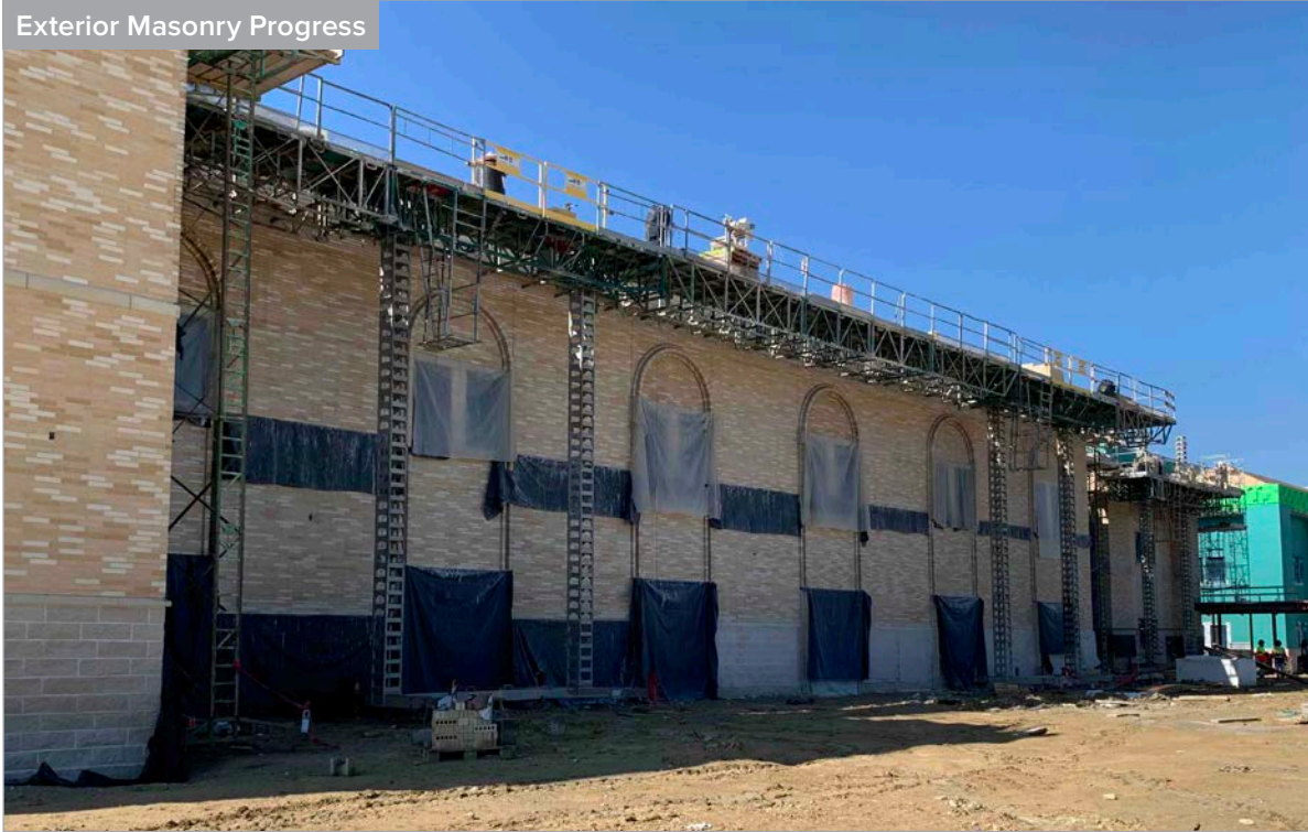
Exterior Masonry Progress
