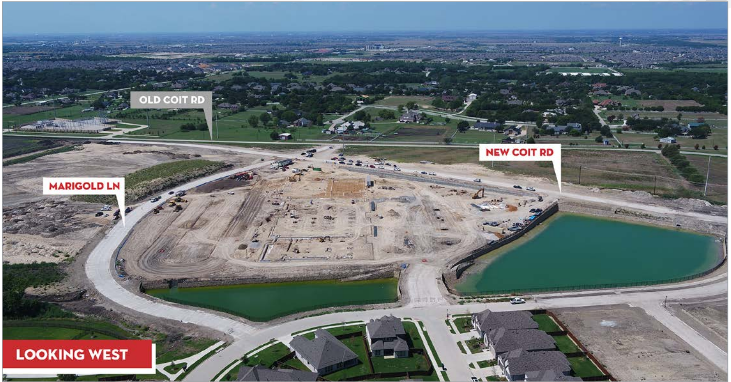
Retaining Wall Foundation and Reinforcing
